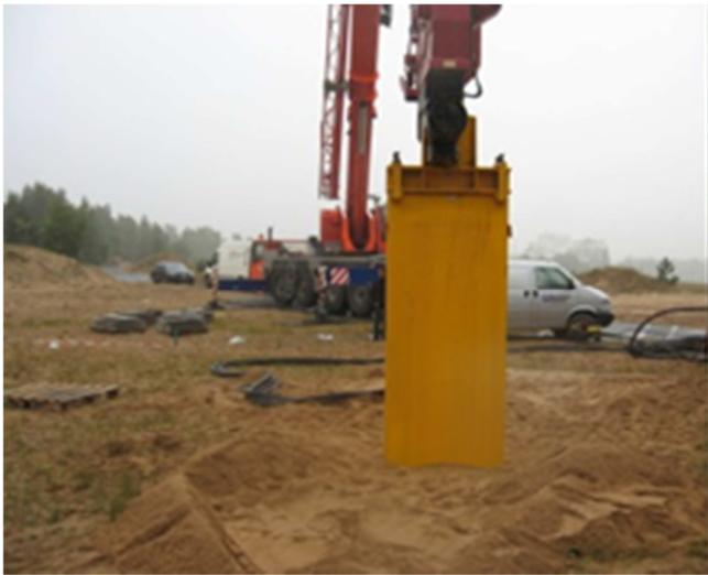
Fig. 6a Driving of installation box
